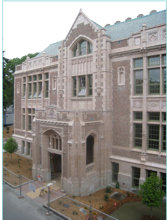
South entrance of the newly renovated Savery Hall. Notice the new landscaping, windows, and the innovative air exchange system on the roof, which combines natural ventilation with variable refrigerant-flow cooling.
